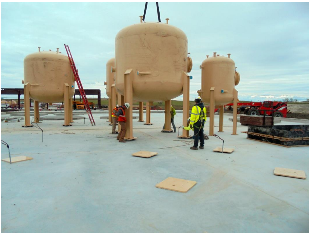
Figure 1: Ion Exchange Columns being installed on site
