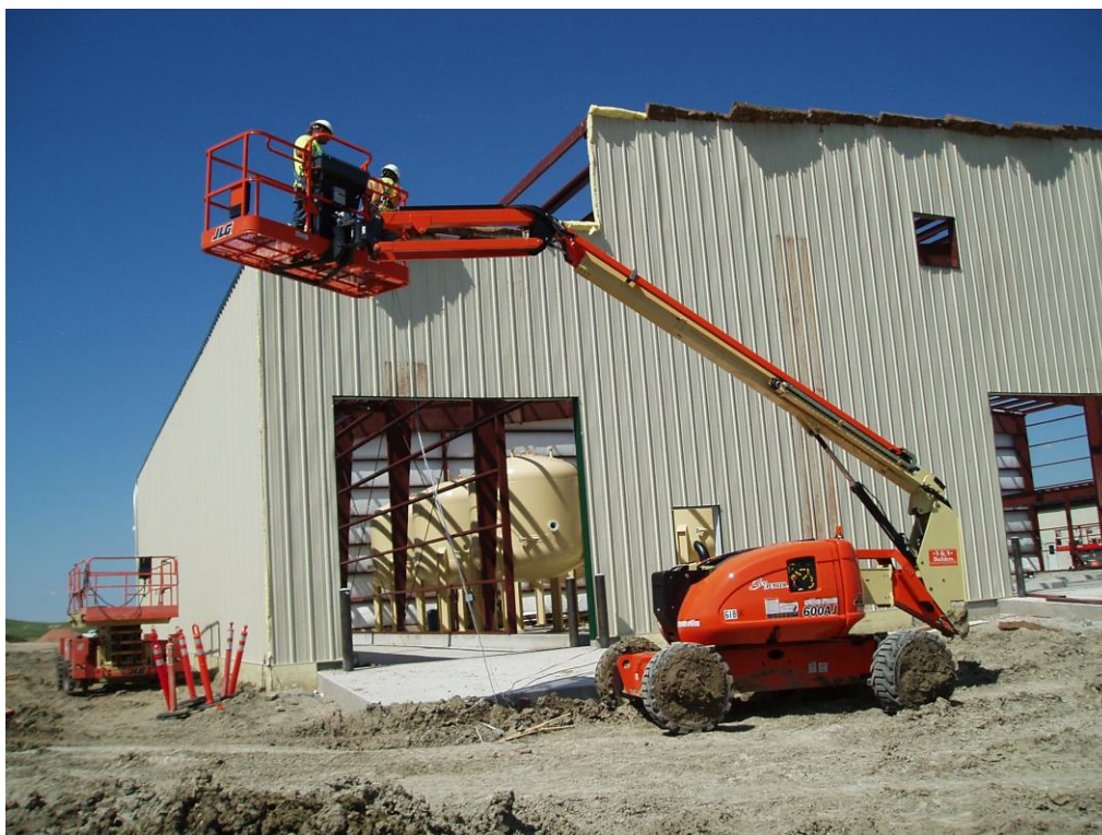
Figure 3: External cladding being fitted to CPP Building
