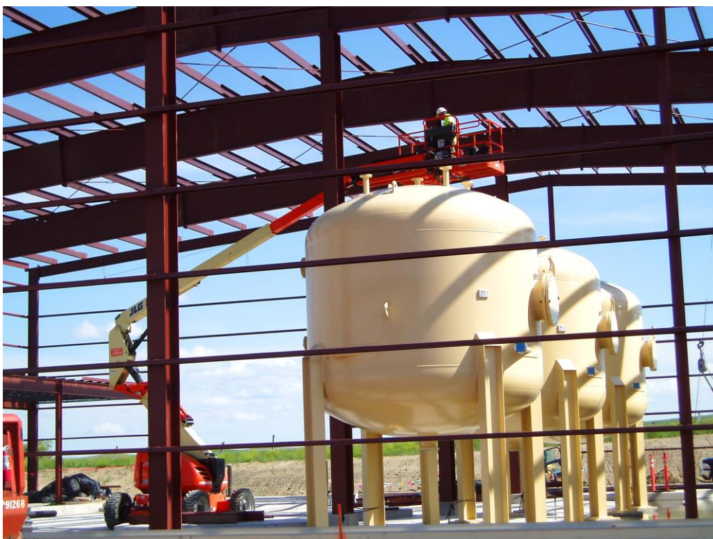
Figure 2: Ion Exchange Columns within the CPP
