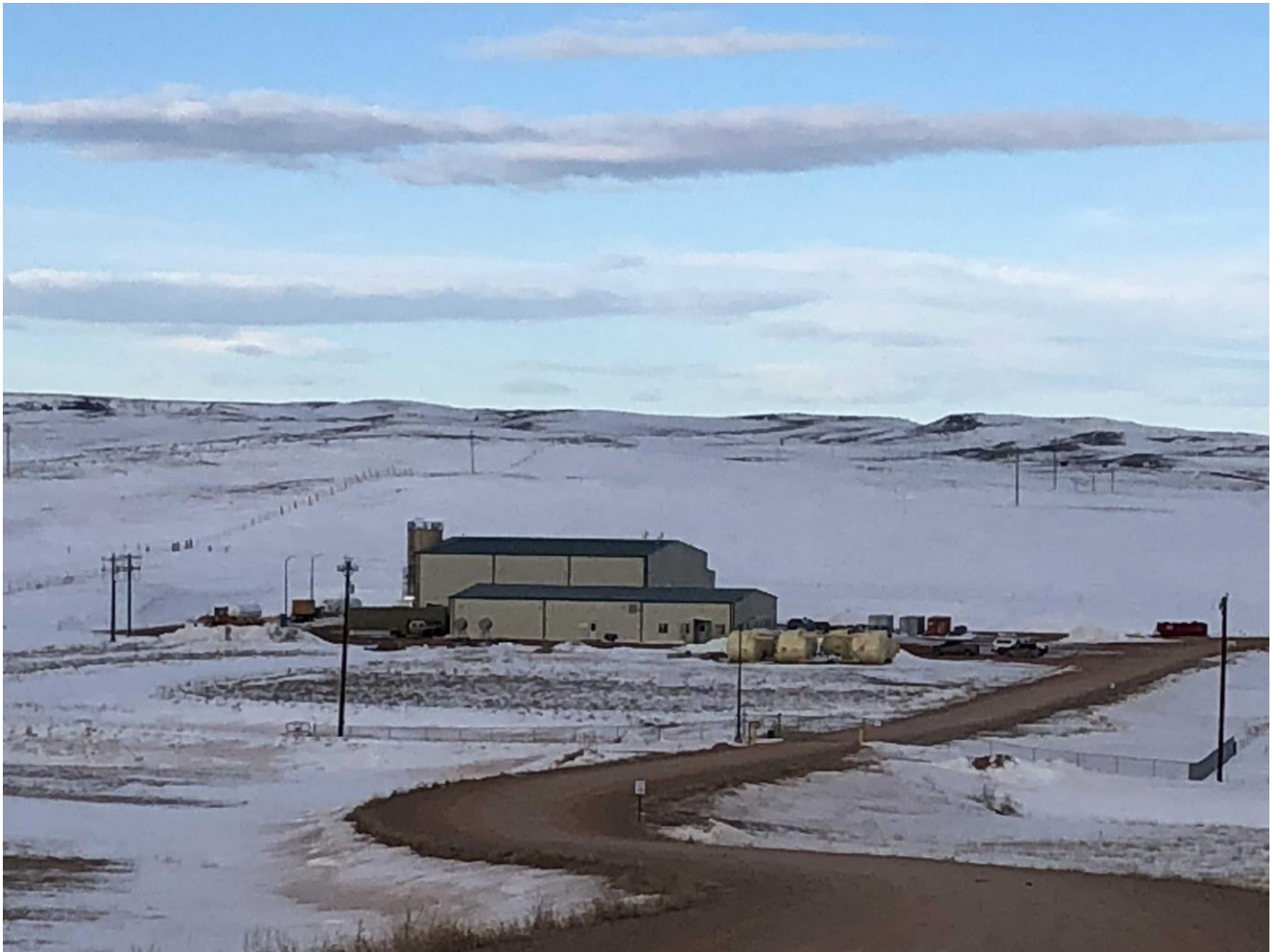
Figure 1: Process Plant and Admin Building, Lance Projects, Wyoming USA (March 2018)
