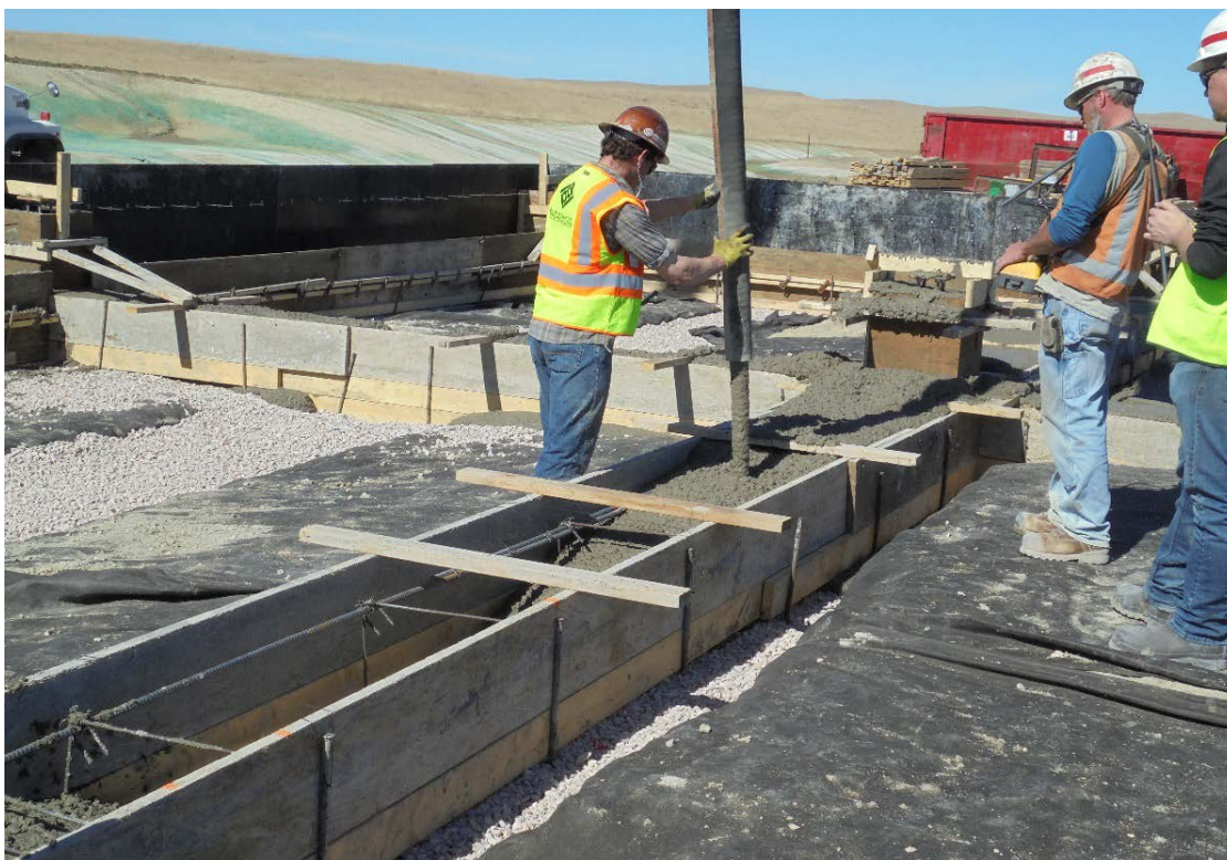
Figure 2: Pouring of foundations for CPP
