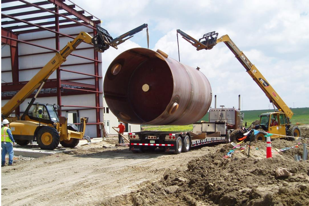
Figure 1: Unloading of tanks at the CPP
