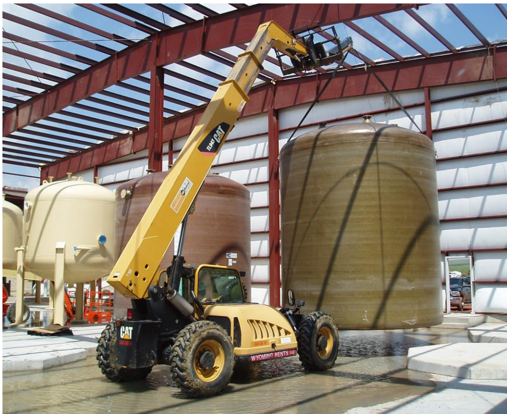
Figure 2: Setting fibreglass tanks inside the CPP
