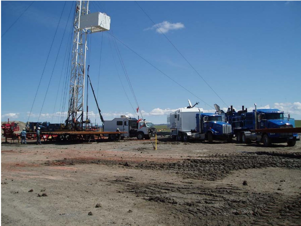
Figure 3: Work-over rig at Deep Disposal Well
