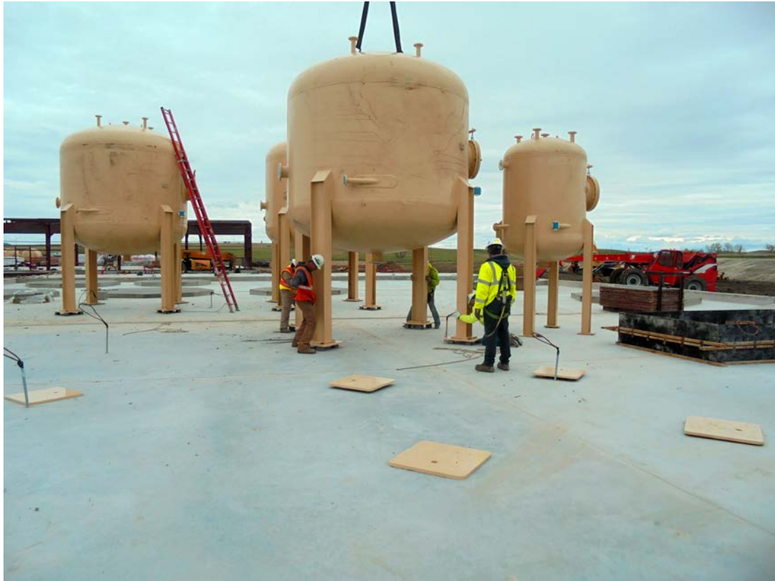
Figure 1: Ion Exchange Columns being installed on site
