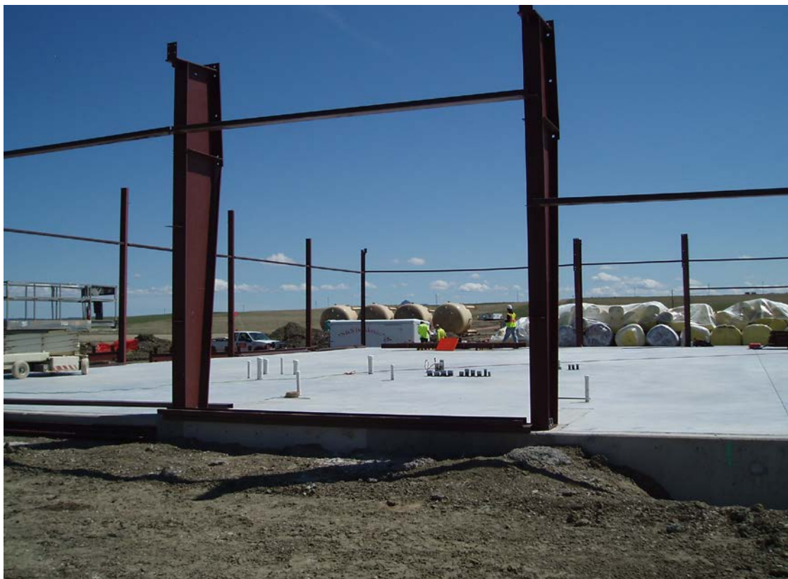
Figure 2: Structural steel erection has commenced
