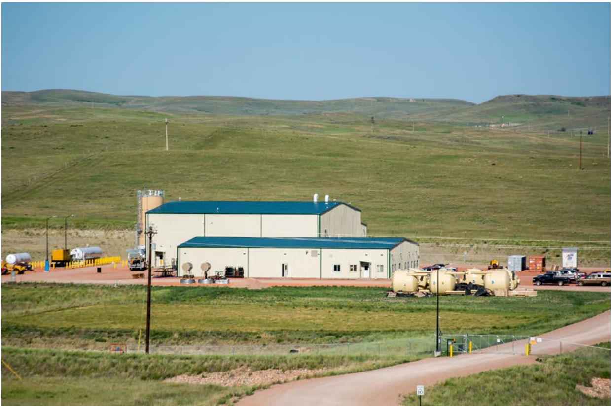
Figure 2: Process Plant and Admin Building, Lance Projects, Wyoming USA
