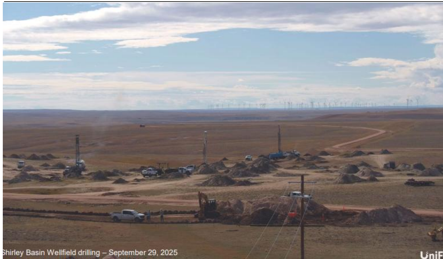
Figure 3: Well field drilling at Shirley Basin
