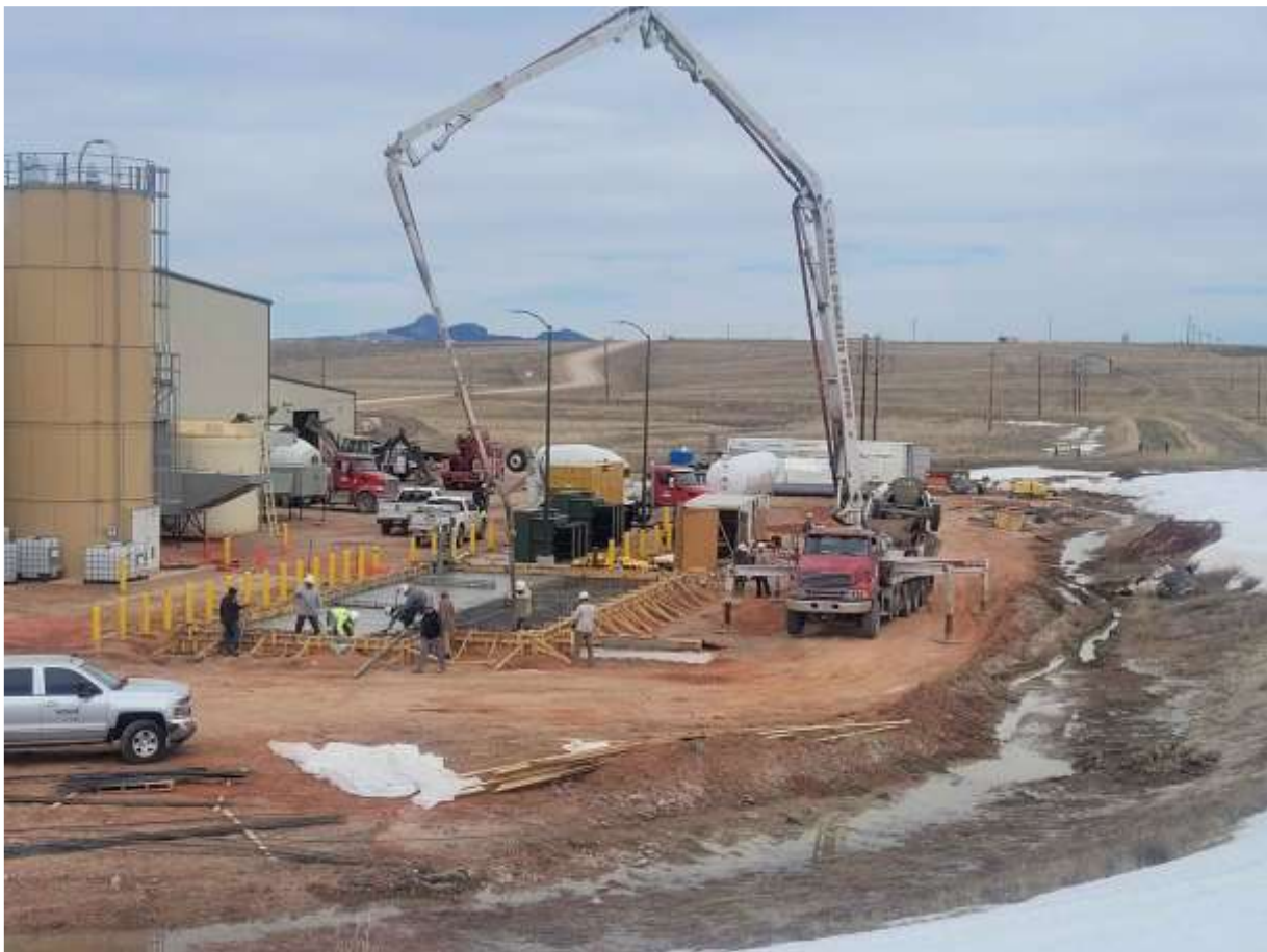
Figure 1: Lance Project, Wyoming USA (concrete foundation pour)
