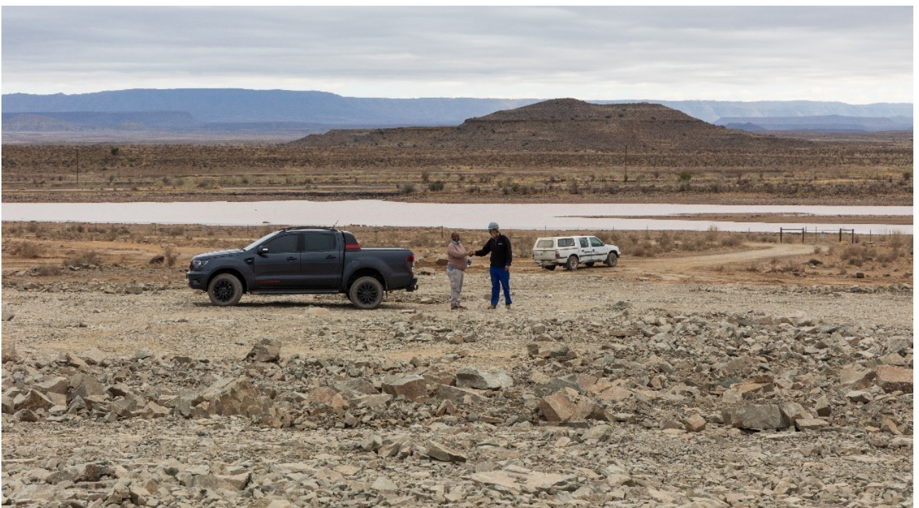
Figure 4-5: Celebrating completion of the backfilling at Rietkuil
