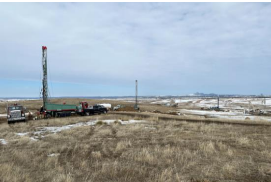
Three contract drilling rigs actively preparing MU-3
