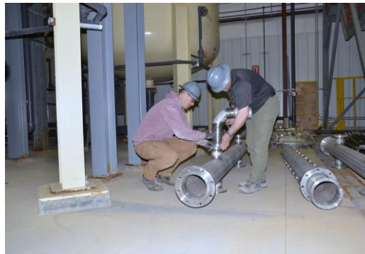
Construction on the process plant nearing completion
