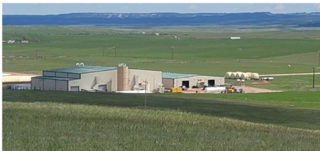
Figure 3: The Ross Process Plant at the Lance Projects, Wyoming USA
