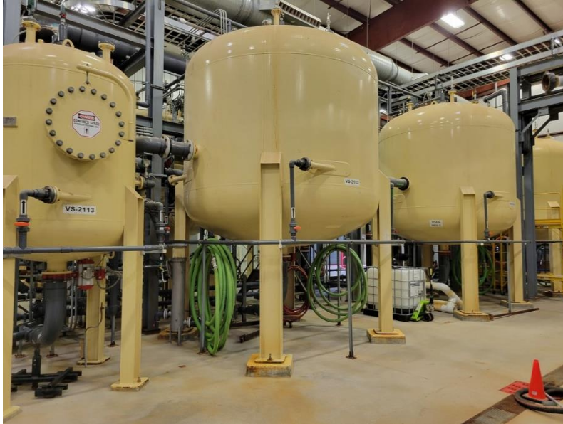
Exhibit 11: Tanks at Lance
