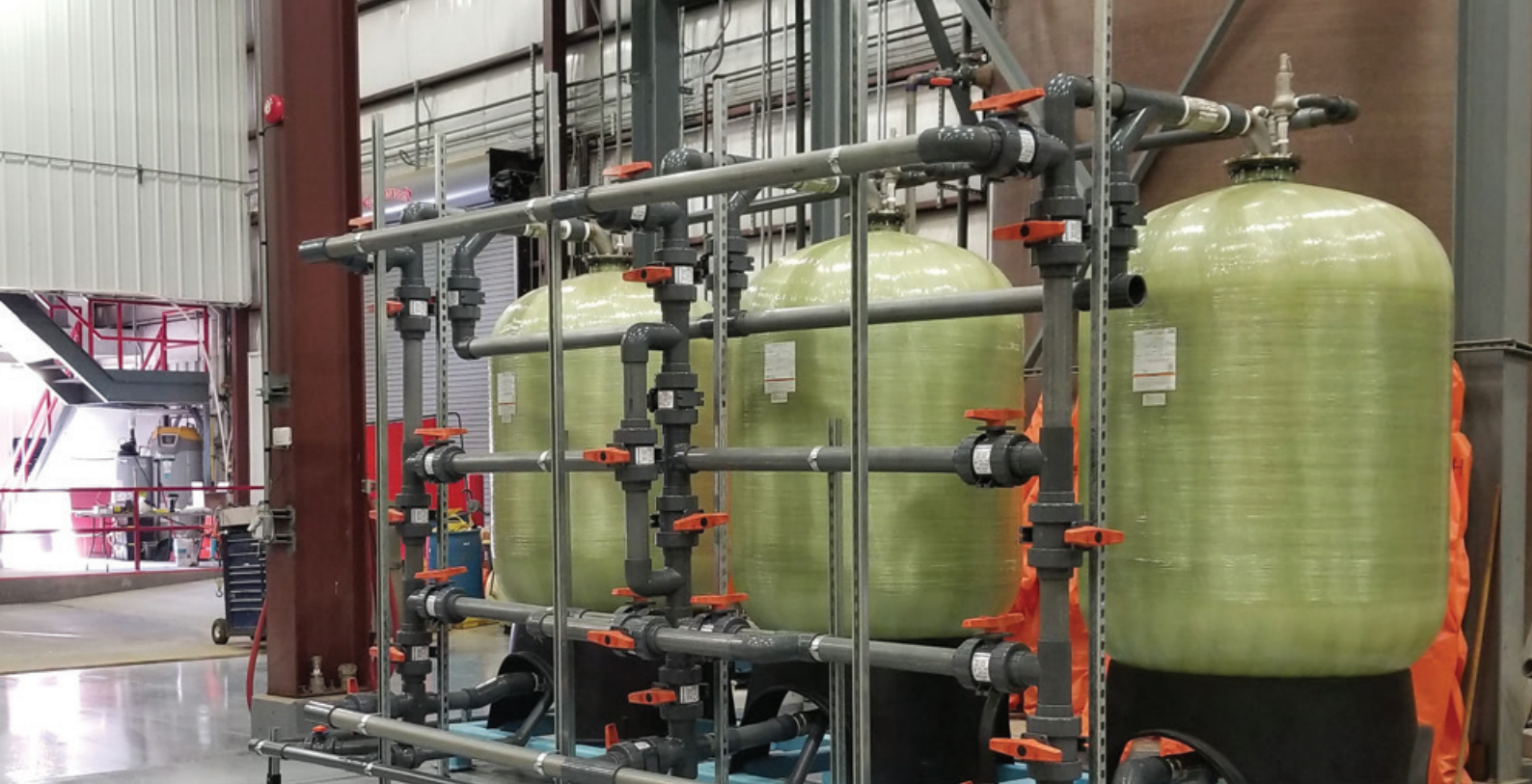
Figure 2: Constructed Ion Exchange Test Columns for MU1A Field Demonstration
