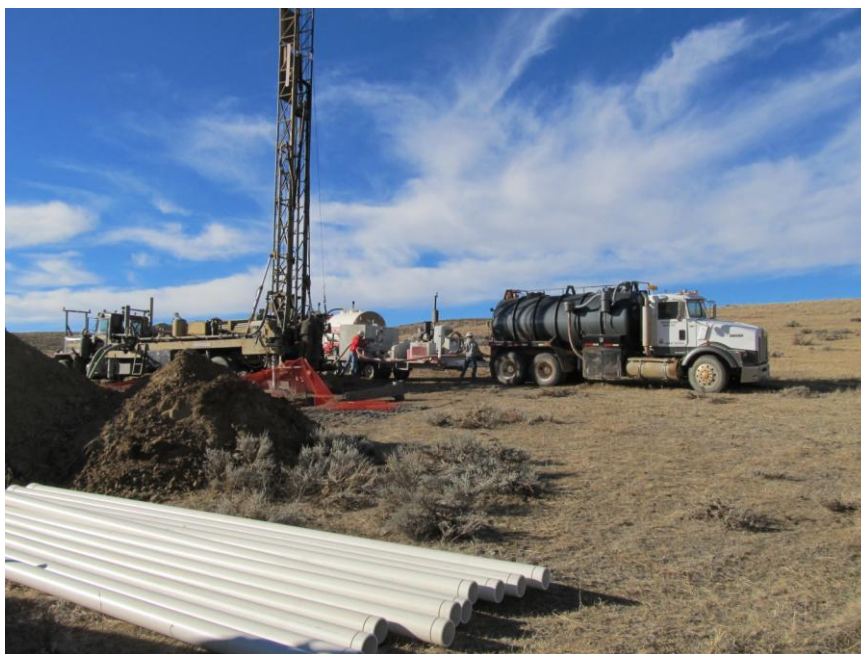
IMAGE 1.4 WELLS ARE DRILLED AT INTERVALS OF 75 FEET / 23 METRES AND AVERAGE DEPTH IS 550-700 FEET / 168-213 METRES
